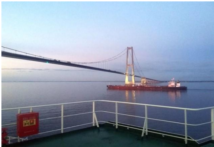
Great Belt Bridge passage
